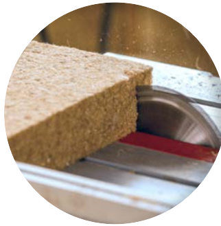
Cutting the Insulation
