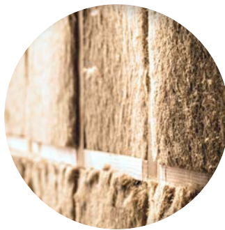
Installing Between Studs
